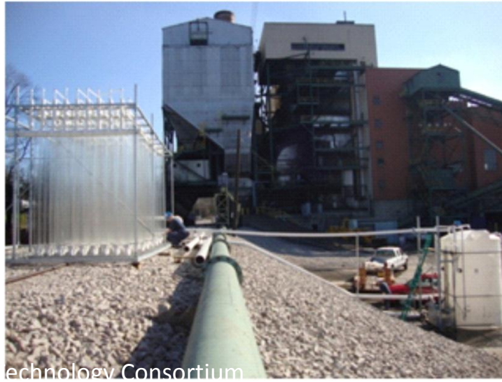
Photobioreactor under construction at Dale Power Station in Kentucky
